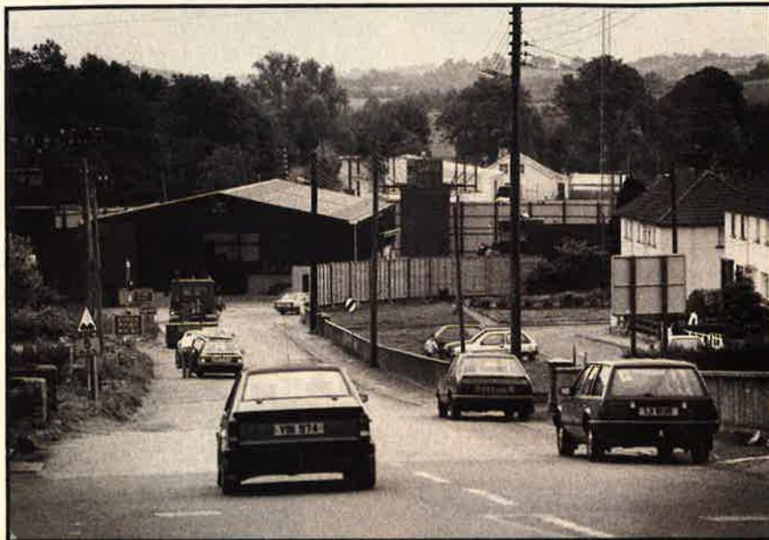
The British Army checkpoint near the Coronation Park housing development
